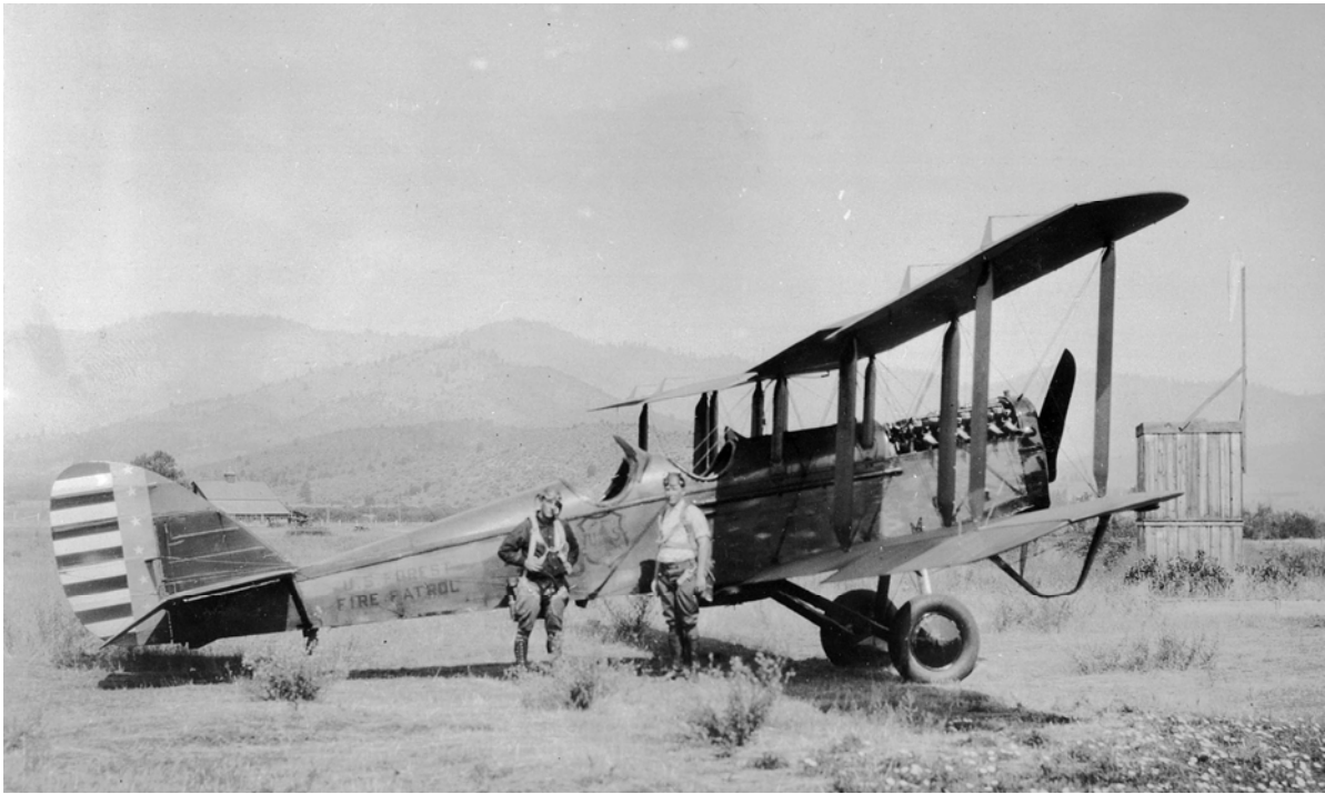
This 1919 photo of an Army Air Service DeHavilland DH-4B shows the first proud use of the Forest Service name on an airplane. The USFS insignia is under the rear cockpit and the large letters U. S. FOREST FIRE PATROL are on the rear of the fuselage. (USFS Photo)
