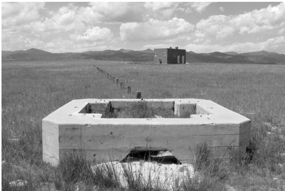
Antenna tower base and central building of the Whitehall, Montana, Low-Frequency Range. Note the line of cable support posts.
