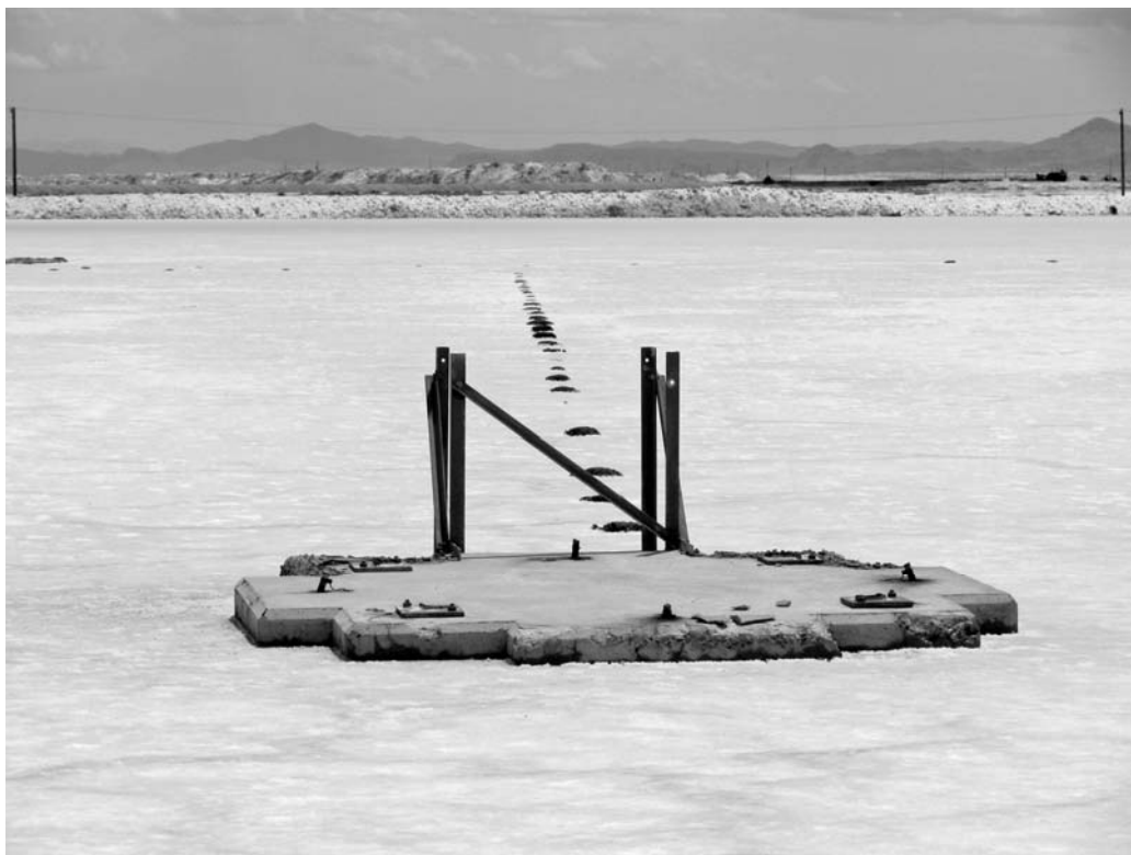
Antenna tower base of the Wendover, Utah, Low-Frequency Range on the salt flats.
